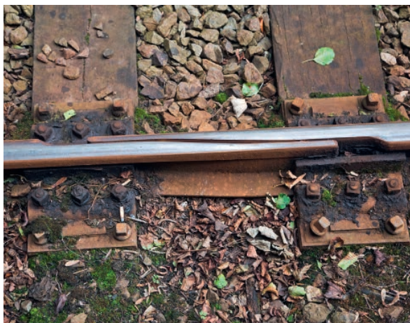
▲ Figure 2.2.4a Tapered overlap of rails
