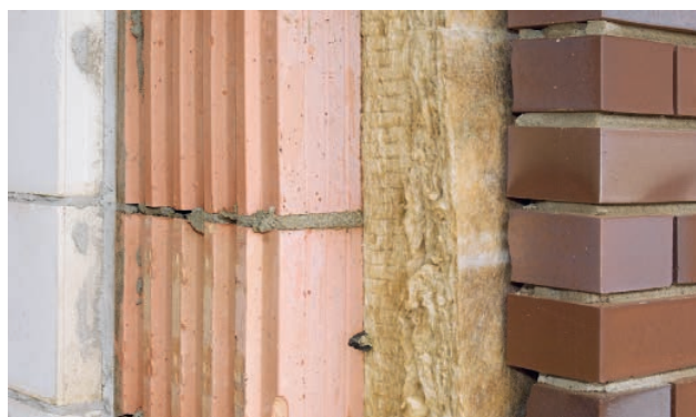
▲ Figure 2.3.12a Foam or wool in a cavity wall provides extra insulation.
