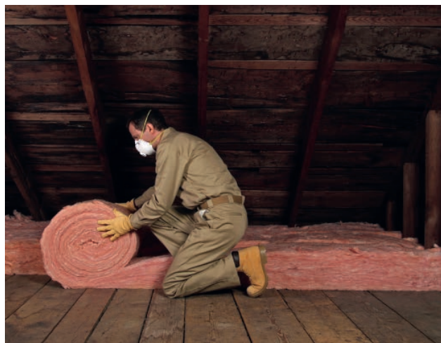
▲ Figure 2.3.12b A thick layer of thermal insulation reduces energy loss through the roof of a building.
