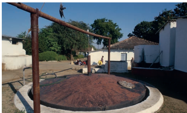
▲ Figure 1.7.18 Methane generator in India
