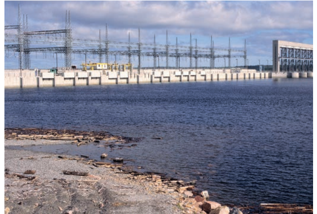
▲ Figure 1.7.16 Tidal barrage in Canada
