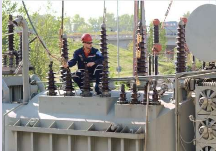
Figure 27.1: This engineer is working on a transformer used for increasing (stepping-up) the size of the alternating voltage to help with the transportation of electrical energy.
