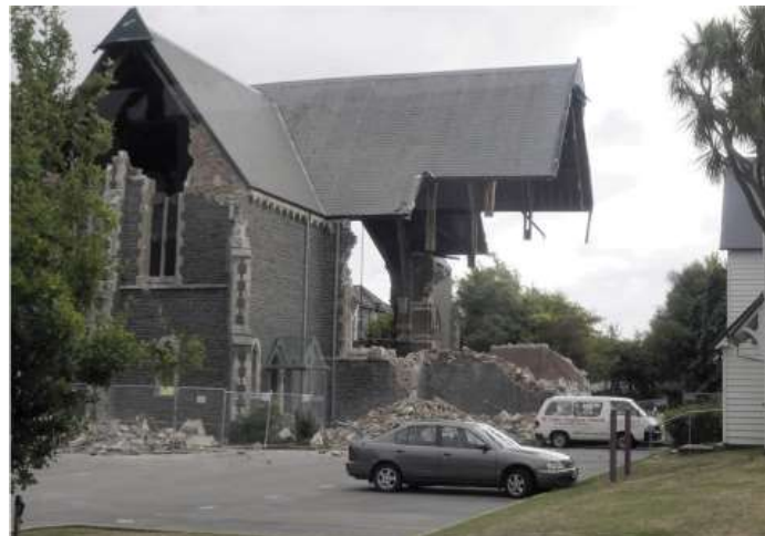
Figure 18.33: Resonance during the Christchurch, New Zealand, earthquake of 22 February 2011 caused the collapse of many buildings. The earthquake, whose epicentre was in Lyttelton, just 10
