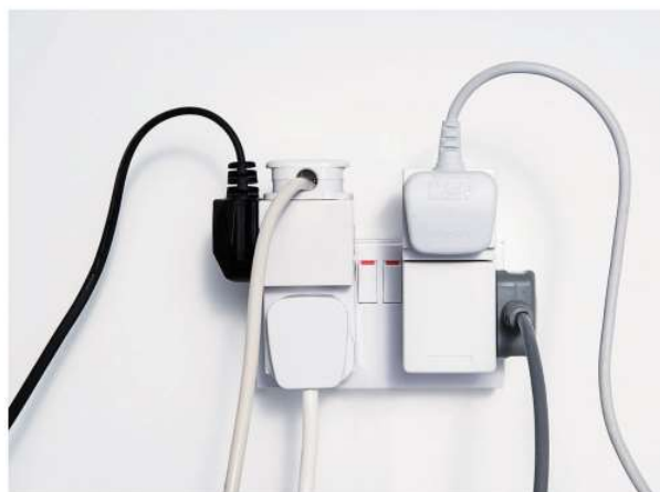
Figure 9.19: a Correct use of an electrical socket. b Here, too many appliances (resistances) are connected in parallel. This reduces the total resistance and increases the current drawn, to the point where it becomes dangerous.
