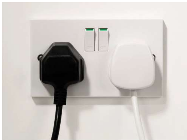
Figure 9.19: a Correct use of an electrical socket. b Here, too many appliances (resistances) are connected in parallel. This reduces the total resistance and increases the current drawn, to the point where it becomes dangerous.
